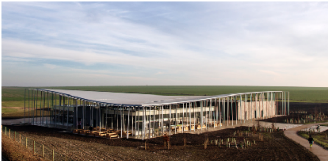
Figure 1. Denton Corker Marshall Visitor Center built for the UNESCO World Heritage site Stonehenge.
